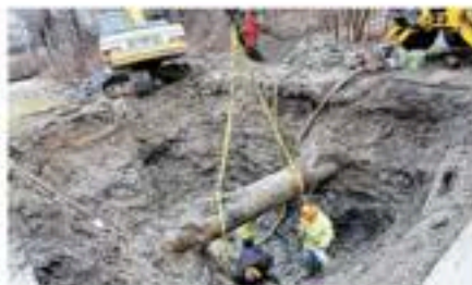
A water main break is repaired in Niskayuna in 2016. Water and sewer jobs are among the hardest for towns to fill. Cindy Schultz/Times Union
